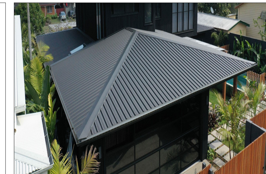
3. COLORBOND MONUMENT METAL ROOF
