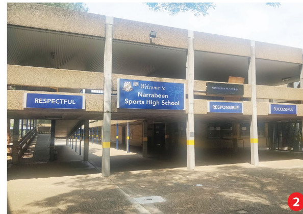
North-eastern corner of Building A
