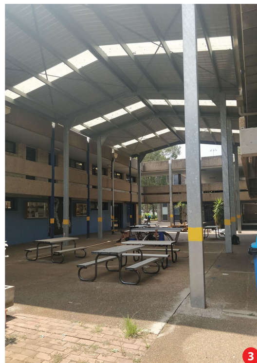
Existing covered courtyard within Building A
