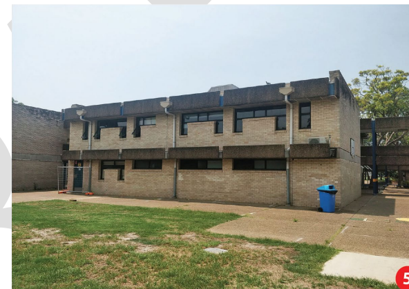
South-western corner of Building A
