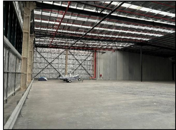
Figure 19. Internal view of warehouse from south-west corner, facing north.
