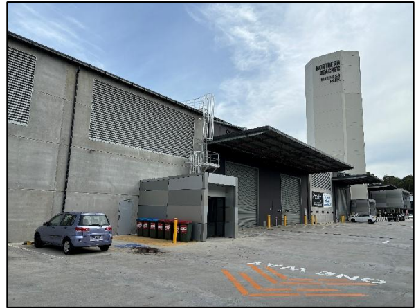
Figure 9. External view of subject site, facing north-west. Note Hexagonal Tower to the right.
