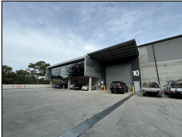
Figure 8. External view of subject site, facing south-west, cantilevered office in view.
