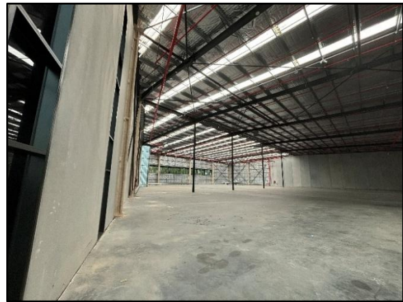
Figure 15. Internal view of warehouse from south-east corner, facing east.
