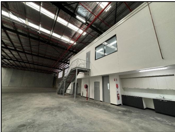
Figure 14. Internal view of warehouse, facing north-east towards office area.
