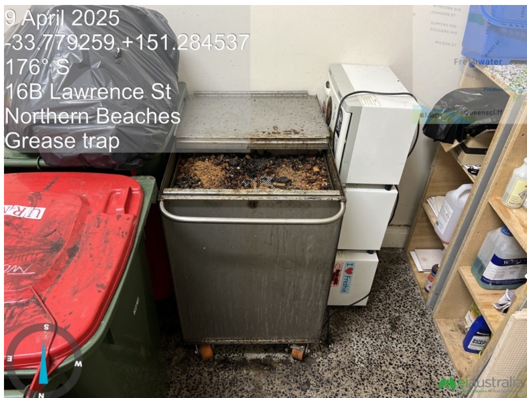
Photograph 6: Facing south, above ground grease trap located in the garbage room at base of pedestrian access stairs from above rooftop carpark.
