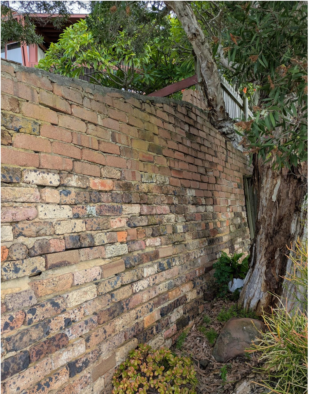
Figure 1: Image of the current masonry retaining wall showing significant erosion of mortar, and a number of large cracks within the wall. Wall shown also in close proximity to tree preventing works.
