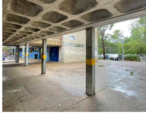
Figure 35: Waffle slab in Main Entry
