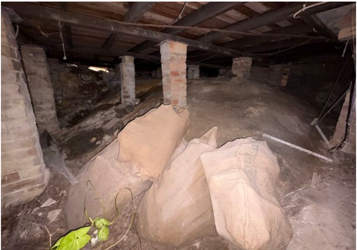
Plate 7: brick pier footings into natural slope below existing dwelling.
