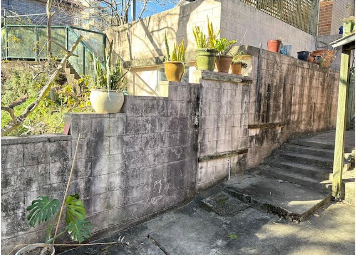
Plate 4: Eastern site boundary with concrete block wall boundary fence.
