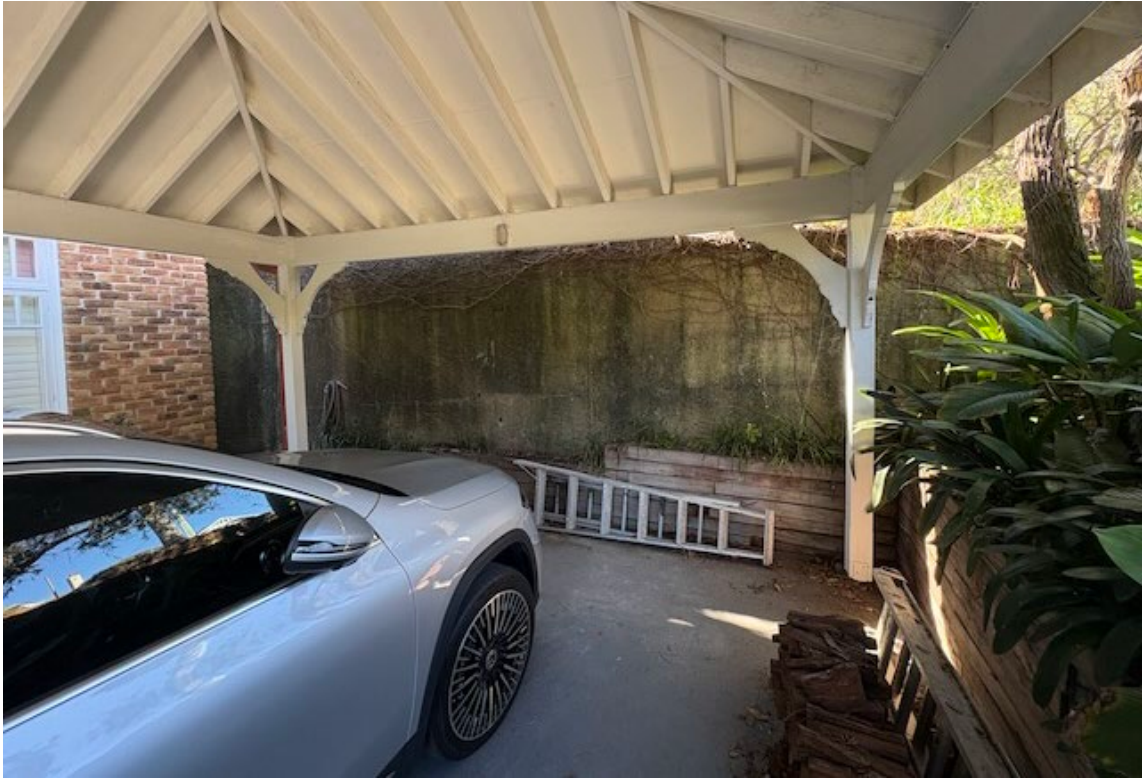
Plate 10: Concrete retaining wall along front southwest boundary with No.40.
