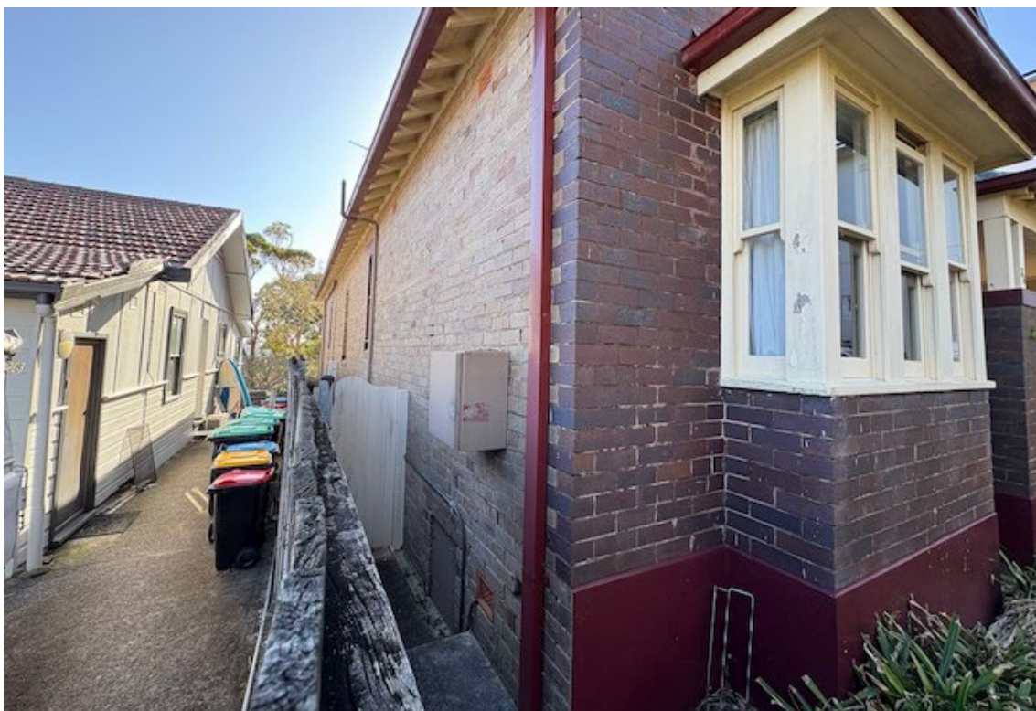
Plate 2: Eastern site boundary viewed to north.
