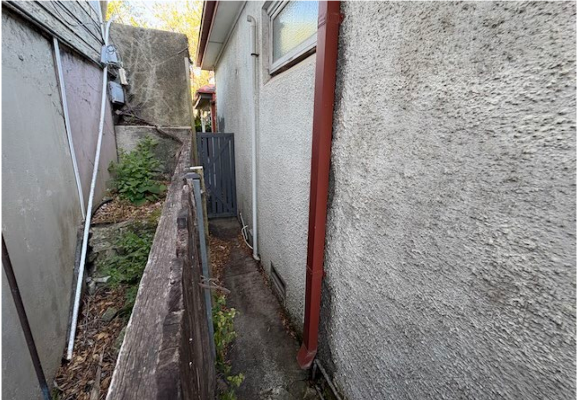
Plate 8: Retained slope, front southwest corner of existing dwelling.
