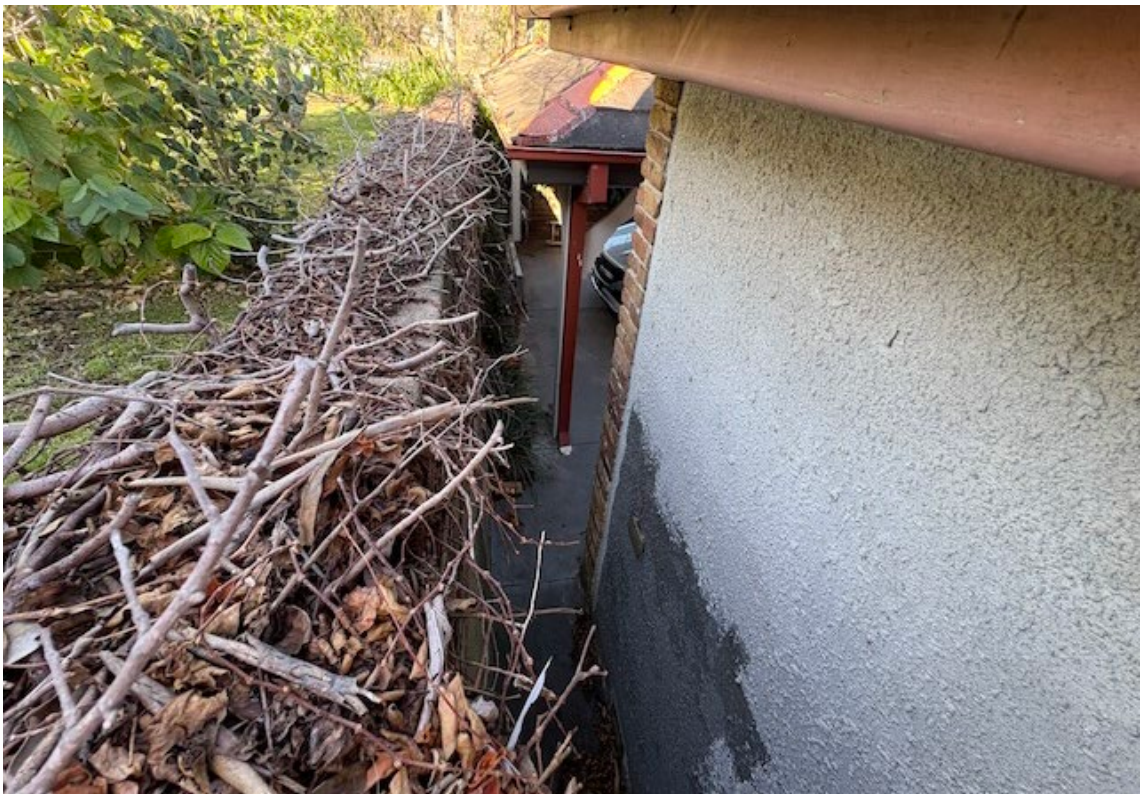
Plate 9: Concrete retaining wall along front southwest corner of site.
