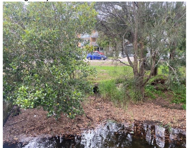
Figure 45: View north towards approximate works area showing drainage culvert and regrowth vegetation along Manly Creek
