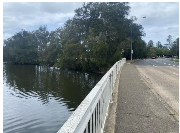
Figure 43: View south along existing pedestrian footbridge crossing Manly Creek
