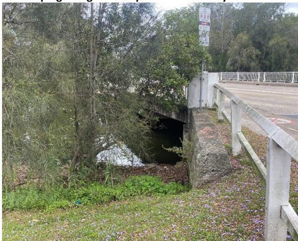
Figure 44: View south-west showing concrete footings of existing pedestrian footbridge along Pittwater Road and approximate works area
