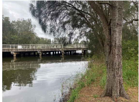
Figure 41: View south-west showing regrowth trees lining Manly Creek, existing pedestrian footbridge and approximate works area
