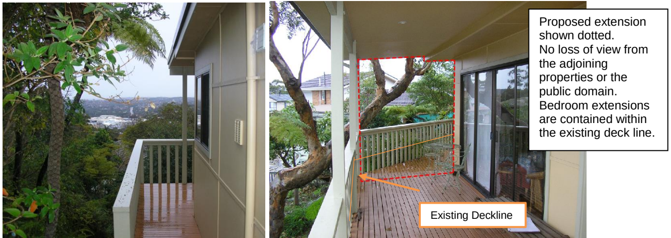
Figure 4: View out towards Beacon Hill and Waringah Mall captured with extension within deck envelope
