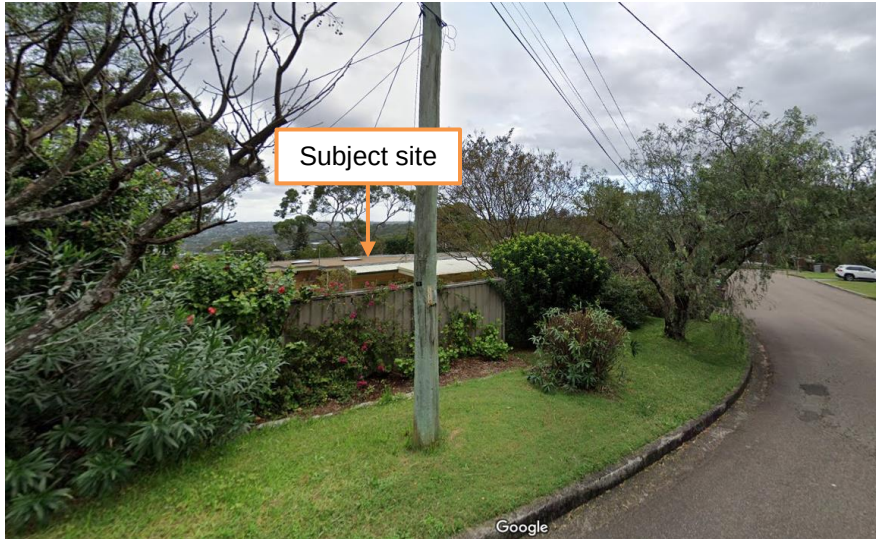
Figure 2: View from Kalianna Crescent showing the front of the site (north). The house sits partially below the street level.
