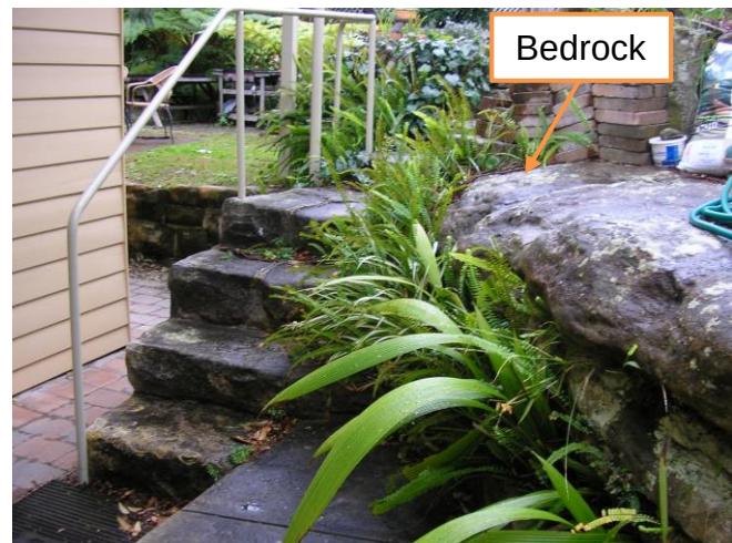
View from Front looking towards the Verandah Area
