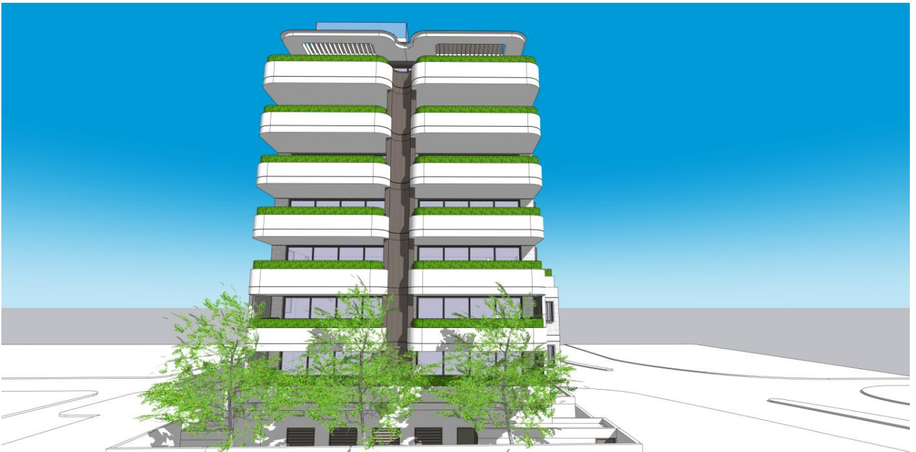
Above: North (rear) façade divided into two vertical forms with recess down the centre of the balconies
