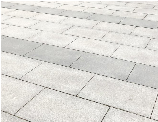
Paving type 2 (P2) - Dark toned sandstone paver
