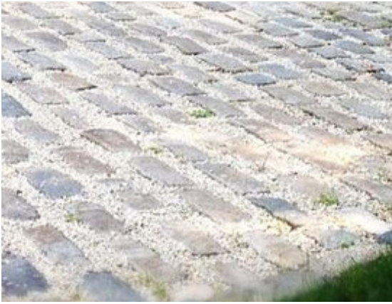
Paving type 3 (P3) - Cobblestone paver
