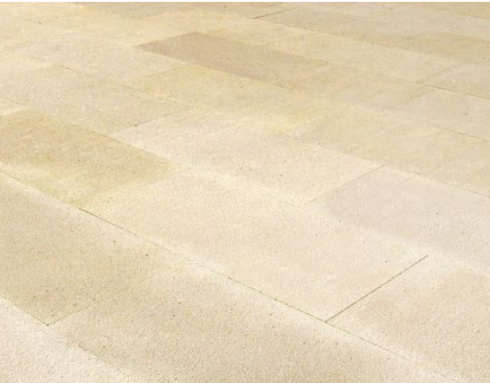
Paving type 1(P1) - Dimensioned sandstone paver
