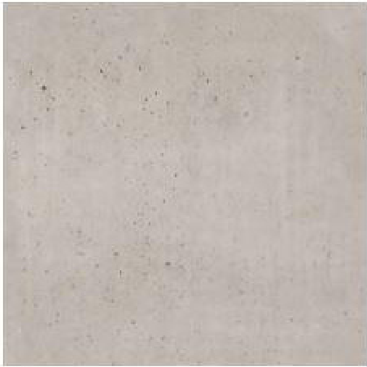
CONC NATURAL OFF-FORM CONCRETE
