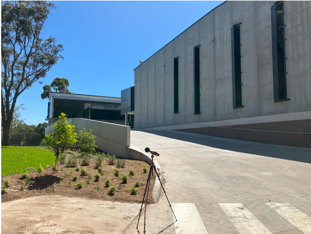
Figure 6: Warehouse external walls are concrete panels with small windows
