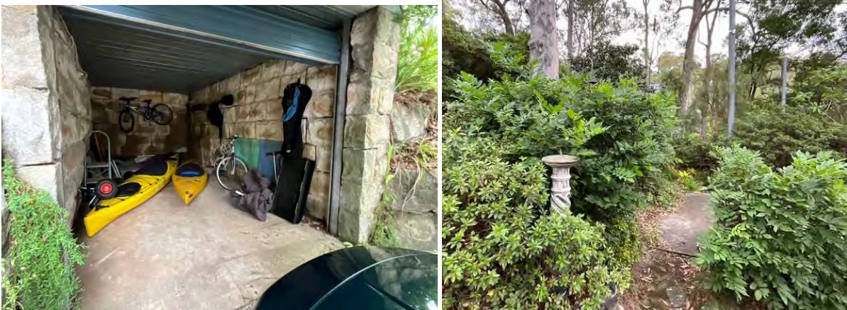
Figures 9 & 10: The existing garage with collapsing sandstone walls (Left) and the roof of the existing garage surrounded by gardens. (Right). (Source: 21 st March 2025).
