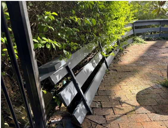
Photograph 5: View of the terrace retaining wall showing signs of rotation, facing northwest
