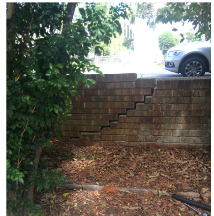
Figure 11—Front fence/retaining wall showing signs of failure. Source: Author
