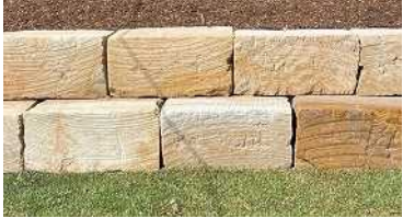
Retaining Wall Sandstone block
