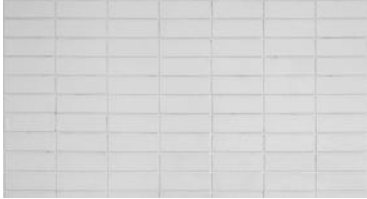
Brick (BWK) Ground Floor External Walls White brick
