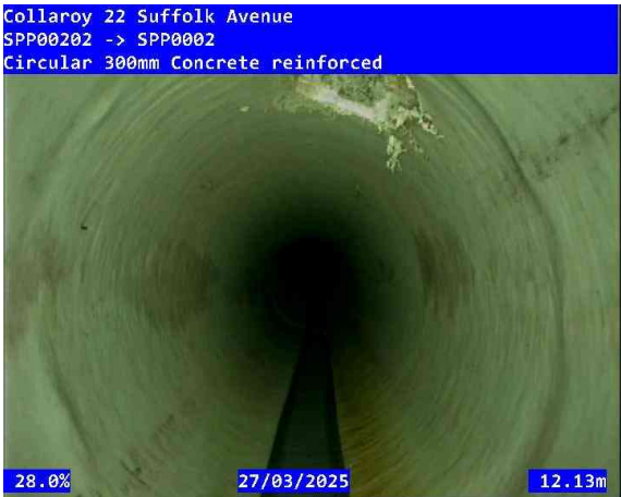
8, 00:06:21, 12.10 Connection, unlined, connection appears to be open, Height/Diameter (mm): 150 at 12 o'clock
