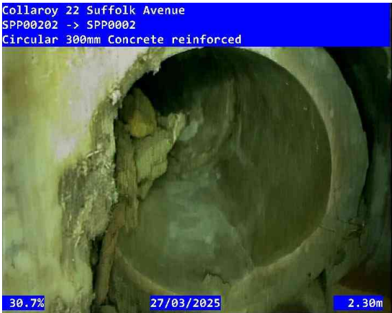
3, 00:03:28, 2.30 Connection, lined, connection appears to be open, Height/Diameter (mm): 150 at 9 o'clock / Possible Pit SPP19823
