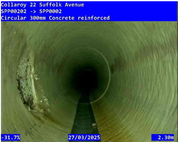
4, 00:03:28, 2.30 Connection, lined, connection appears to be open, Height/Diameter (mm): 150 at 9 o'clock / Possible Pit SPP19823
