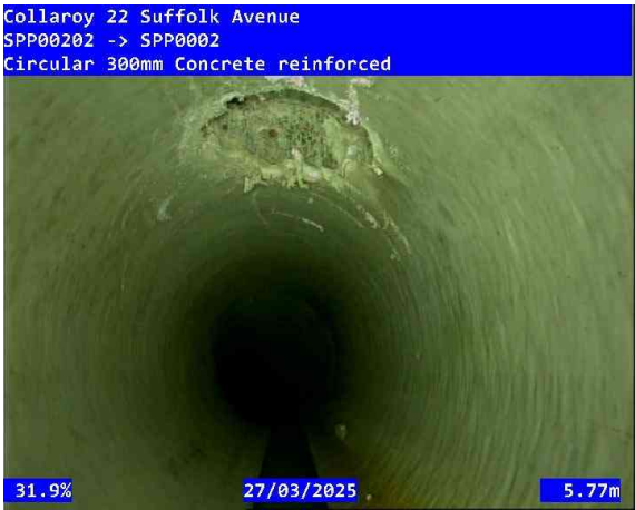
6, 00:04:45, 5.75 Connection, lined, connection appears to be open, Height/Diameter (mm): 150 at 1 o'clock / Possible pit SPP19824
