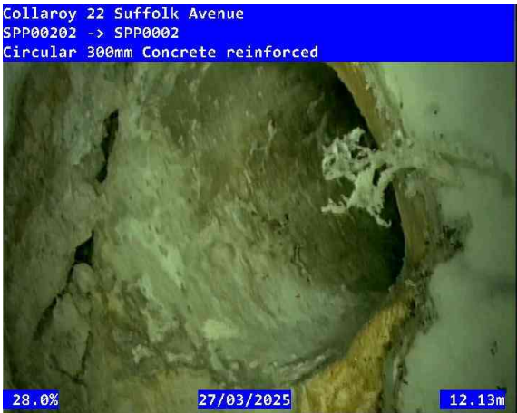
7, 00:06:21, 12.10 Connection, unlined, connection appears to be open, Height/Diameter (mm): 150 at 12 o'clock
