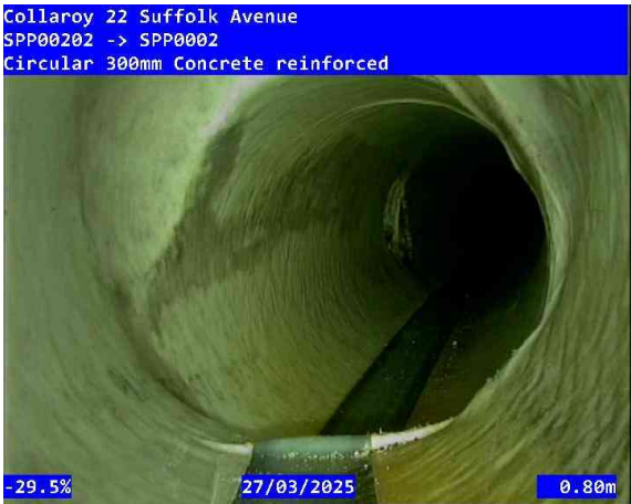
2, 00:02:24, 0.80 Horizontal deformation, change in diameter: 20% at 5 o'clock
