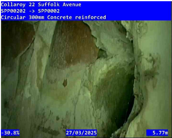
5, 00:04:45, 5.75 Connection, lined, connection appears to be open, Height/Diameter (mm): 150 at 1 o'clock / Possible pit SPP19824
