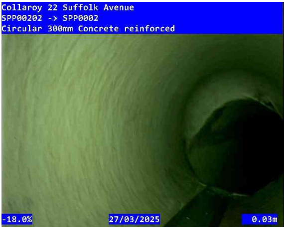
1, 00:00:47, 0.00 Point repair, injected sealing material, length: 1000mm from 12 o'clock to 12 o'clock
