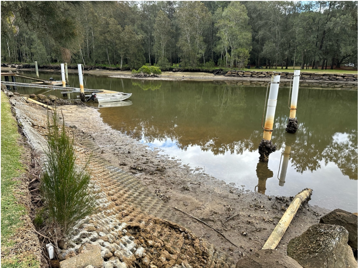
Figure 5 - Existing concrete mesh seawall, storm water pipe and piles with significant degradation and failure of the mesh concrete in the foreground
