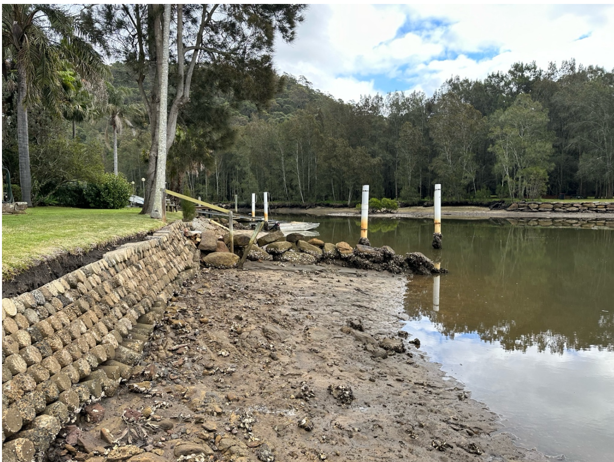
Figure 4 - Existing concrete cylinder seawall and rock groyne with dislocation of concrete cylinders and significant slumping of the soil behind the seawall clearly evident
