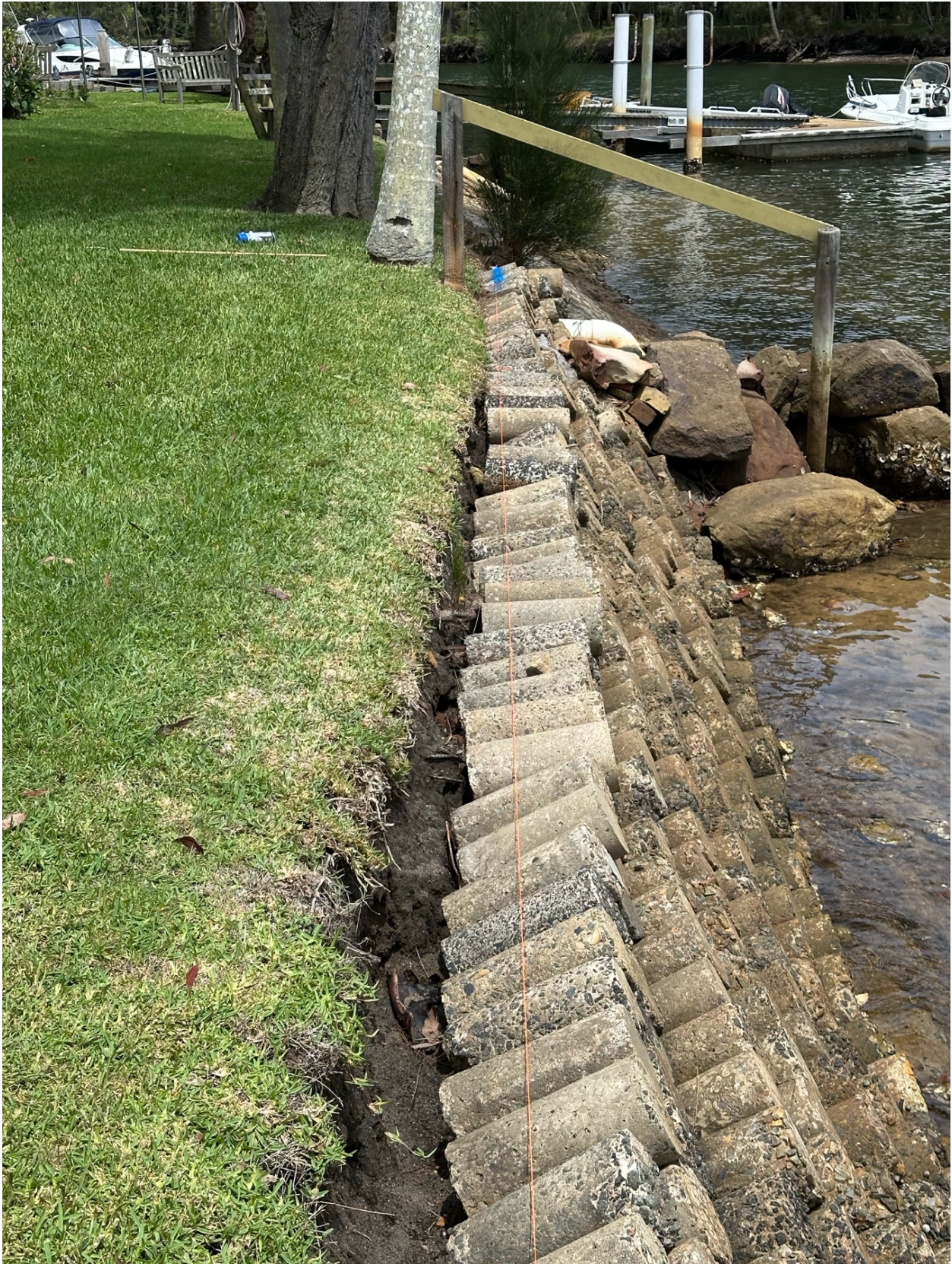
Figure 7 - Significant soil slumping behind concrete cylinder seawall – orange string line depicts surveyed boundary
