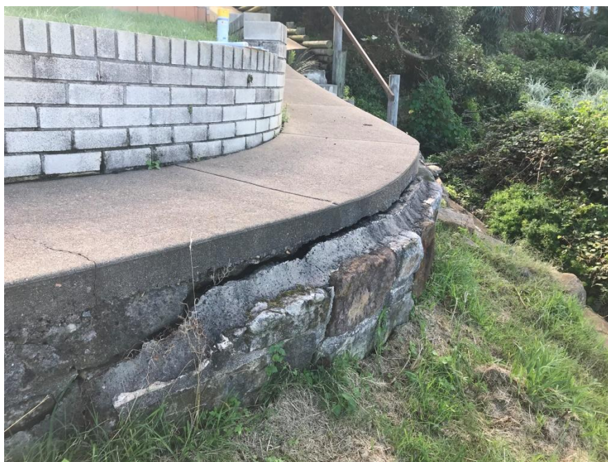
Photograph 5: View of the mortared sandstone retaining wall in the rear of the property.
