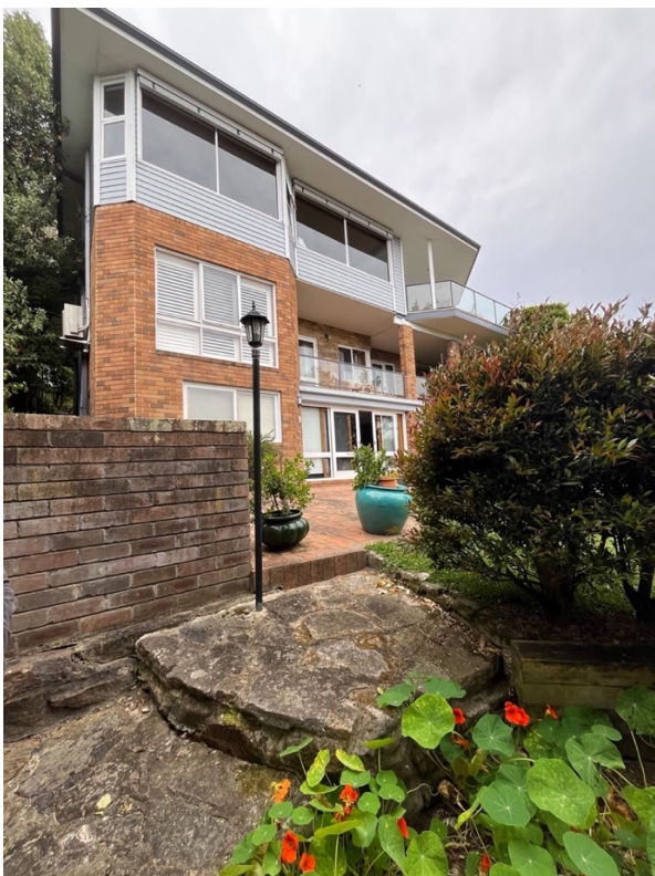
Photo 6 – Rear elevation of existing primary dwelling.
