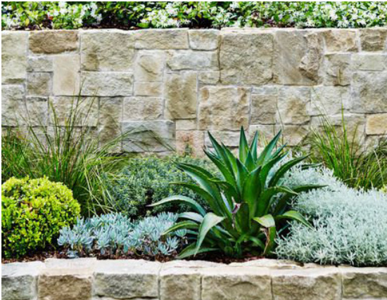
Retaining wall (W) - Sandstone clad wall
