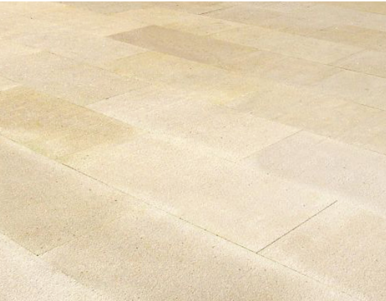
Paving type 1(P1) - Dimensioned sandstone paver
