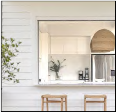
1 - WEATHERBOARD CLADDING: DULUX NATURAL WHITE OR SIMILAR
