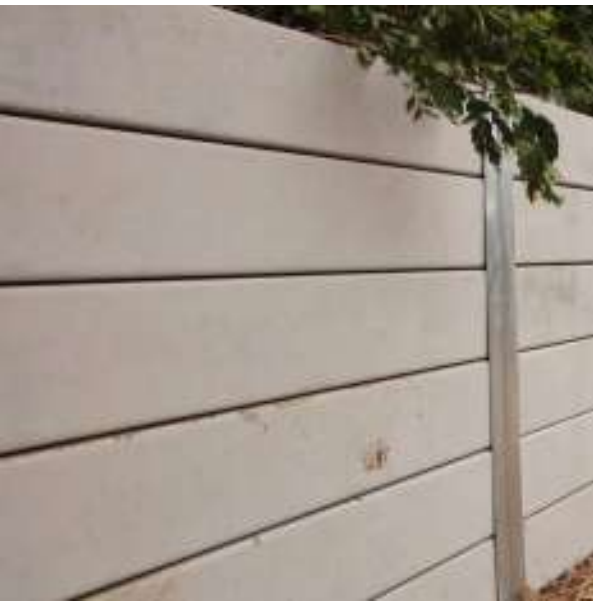
Concrete Sleeper Retaining
