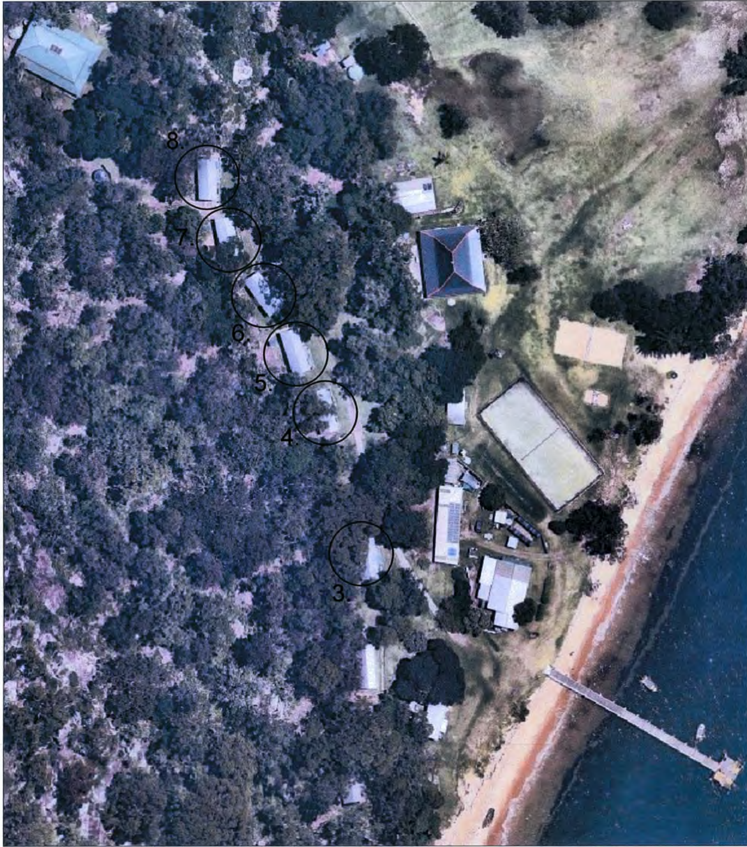
AERIAL PHOTO OF SITE
