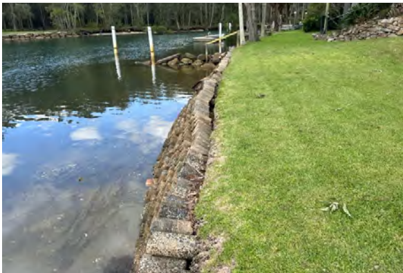
Photo 3: Concrete cylinder seawall in dilapidated condition on western boundary of site. Image showing rock rubble and sediments overlaying bedrock shelf in McCarrs Creek watercourse, photo looking north.
