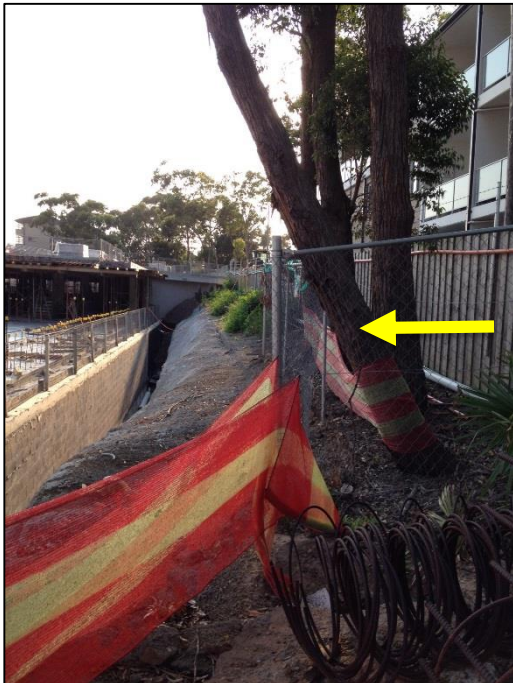
Photo 3: Lean on the tree and adjacent excavation works.
