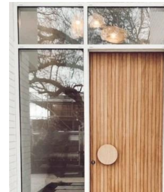
05. CL - V-groove timber cladding. Dulux white or similar
