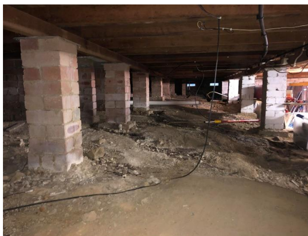
Photograph 9: Exposed footings in basement sub floor level, facing south east
