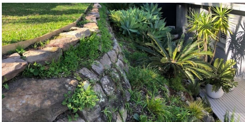
Photograph 5: Lower front retaining wall, facing south east
