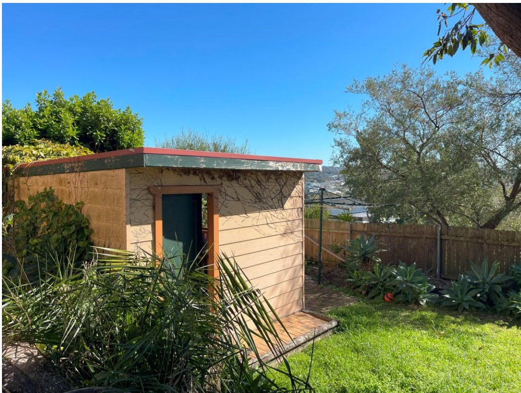
Fig 5: View of the existing rear yard and detached shed (to be demolished), looking north-west
