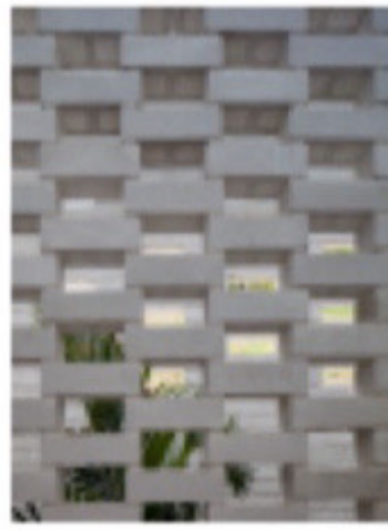
8. HIT AND MISS BRICKWORK
