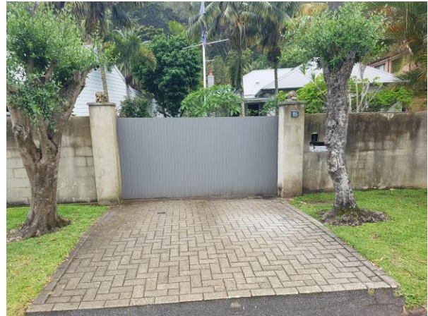
Existing driveway, looking East
