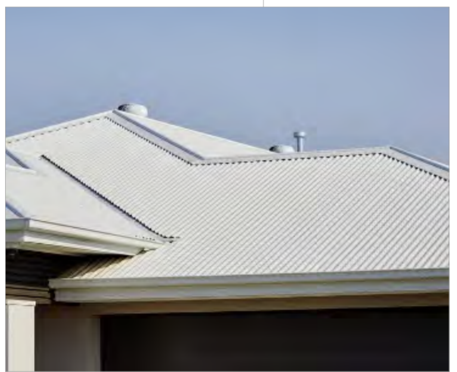
COLOUBOND METAL ROOF SHEETING - FINISH TO BE LIGHT OR SIMILAR TO BE CONFIRMED BY CLIENT
