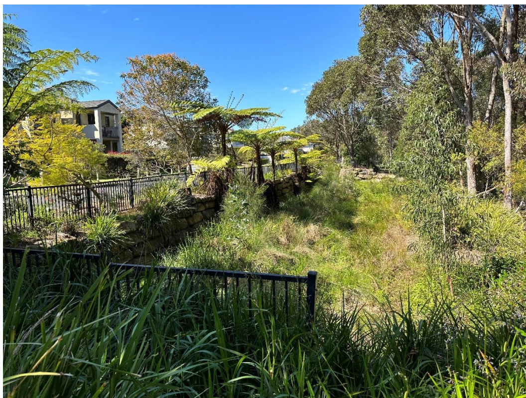
Figure 27: Area F sandstone block retaining wall in riparian corridor.
