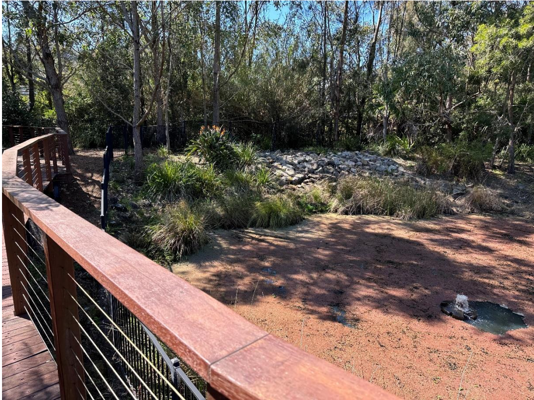
Figure 32: Area G stormwater pond riprap overflow weir.
