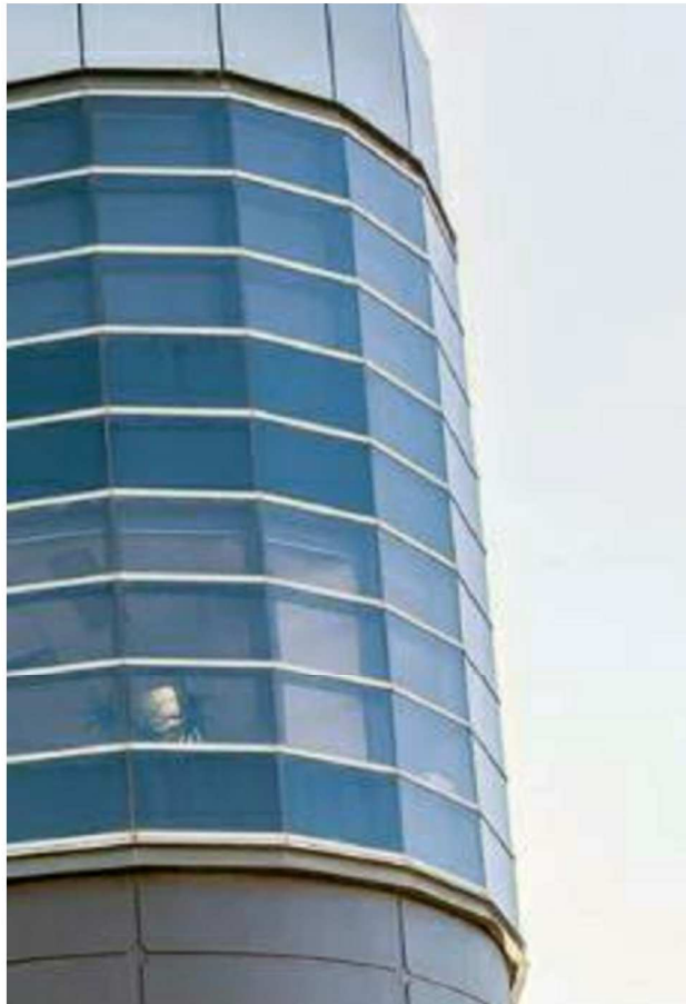
ED-02 CURTAIN WALL MATCH NEIGHBOURING BUILDING WITH A MIXTURE OF DARK TINTED GLASS PANELS (GL-01) AND OPAQUE PANELS (GL-02)
