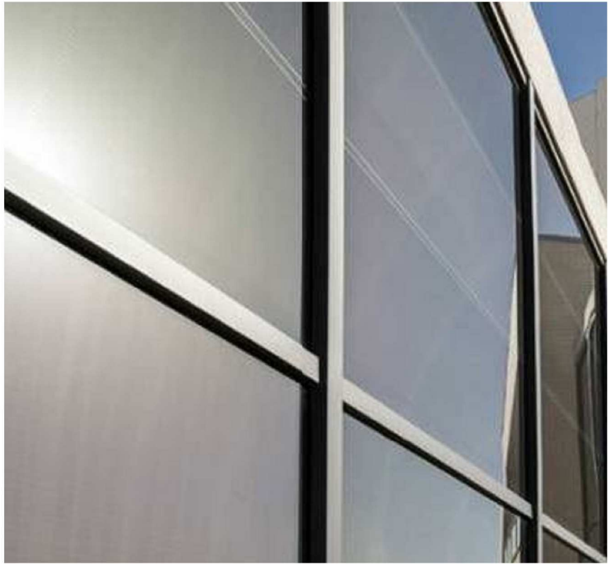
ED-01 CURTAIN WALL WITH A MIXTURE OF DARK TINTED GLASS PANELS (GL-01) AND OPAQUE PANELS (GL-02)
