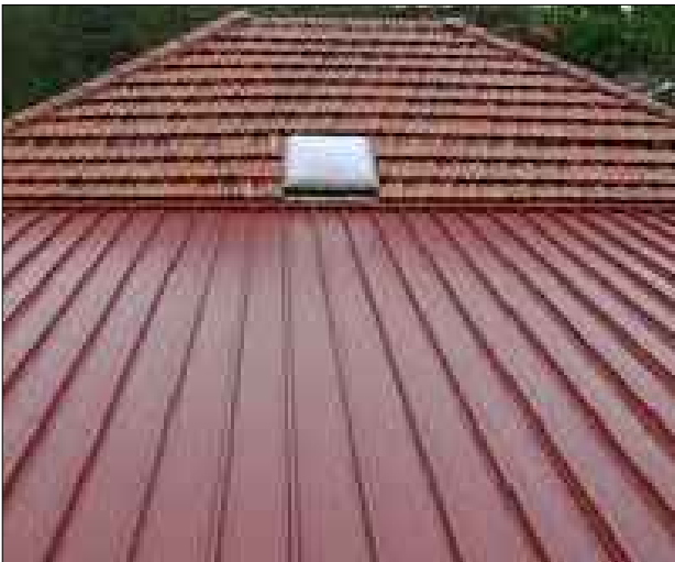
NEW ROOFING: METAL ROOF SHEETING Col. Colorbond Manor Red
