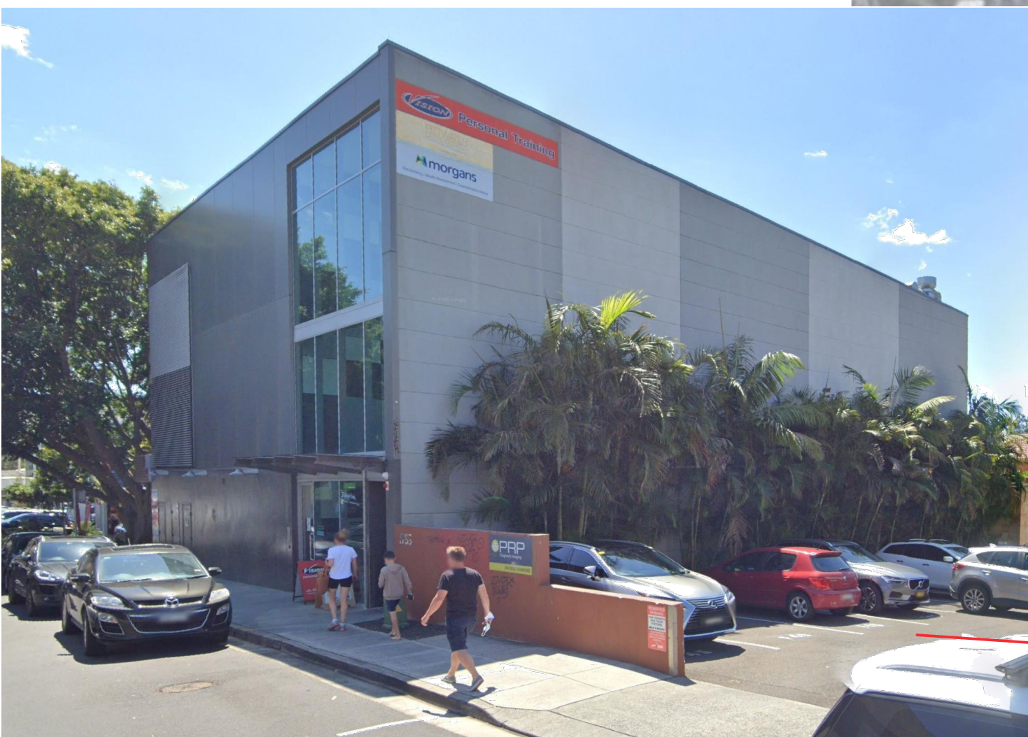
A WARATAH STREET STOREY BUILDING
