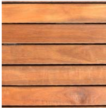
Timber decking & soffits
