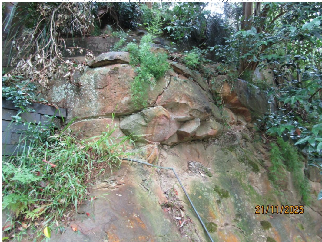
Photo 3– close up of cliff face below proposed spreader, showing cracking.
