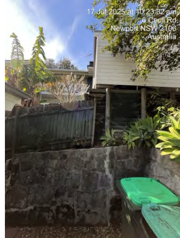
Photo 2: Sandstone flagging wall downslope of adjoining structure footings on the eastern boundary of the subject site
