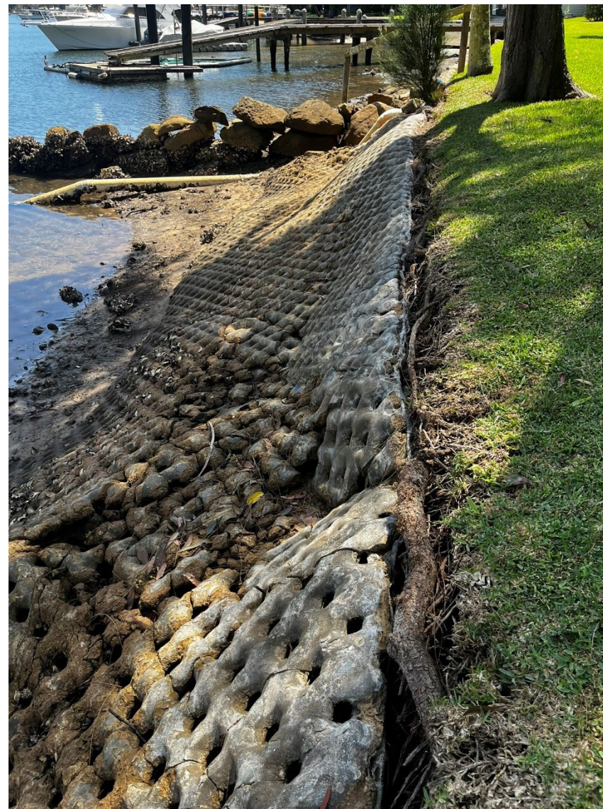
Image 4. Dilapidated Seawall showing casuarina roots along top edge
