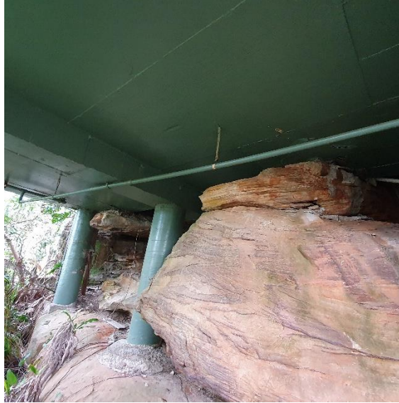
Photograph-7: Concrete piers supporting the pool. View looking up south-east.
