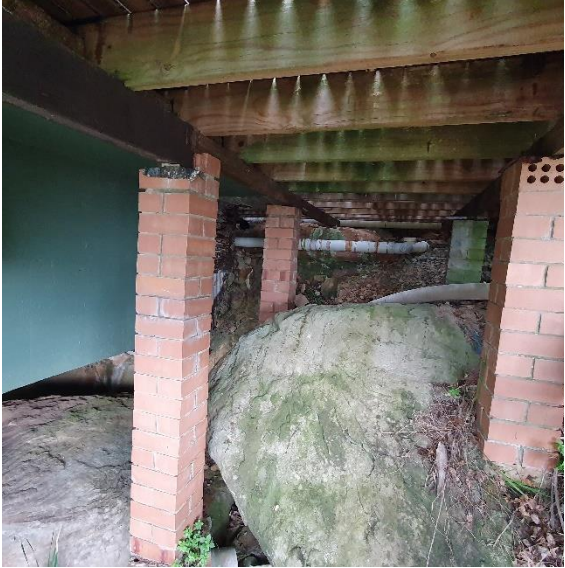
Photograph-6: Brick piers supporting the timber deck. View looking south.
