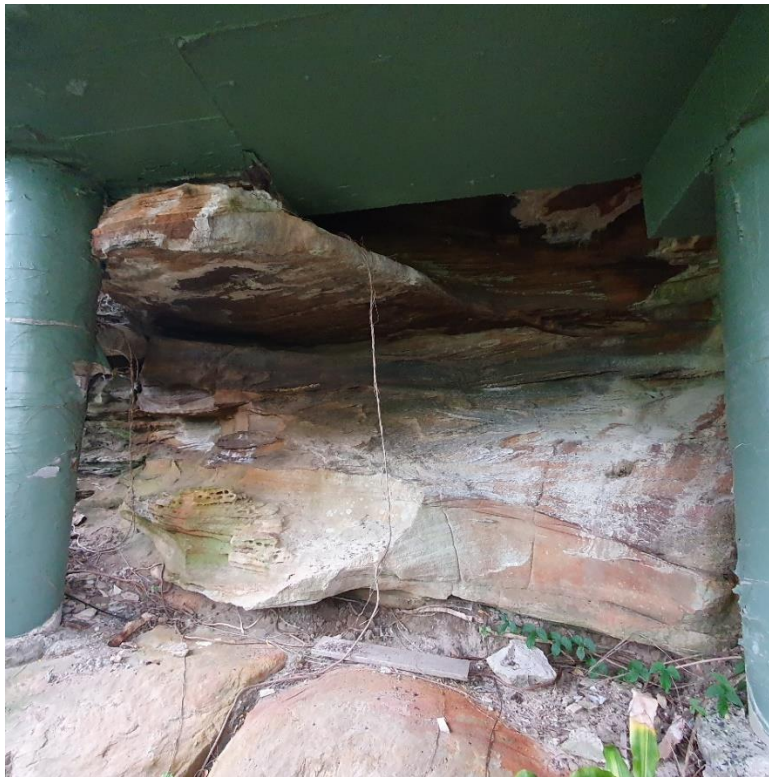
Photograph-8: Sandstone bedrock cliff face below the pool displaying sub-horizontal bedding defects and minor undercutting. View looking south.
