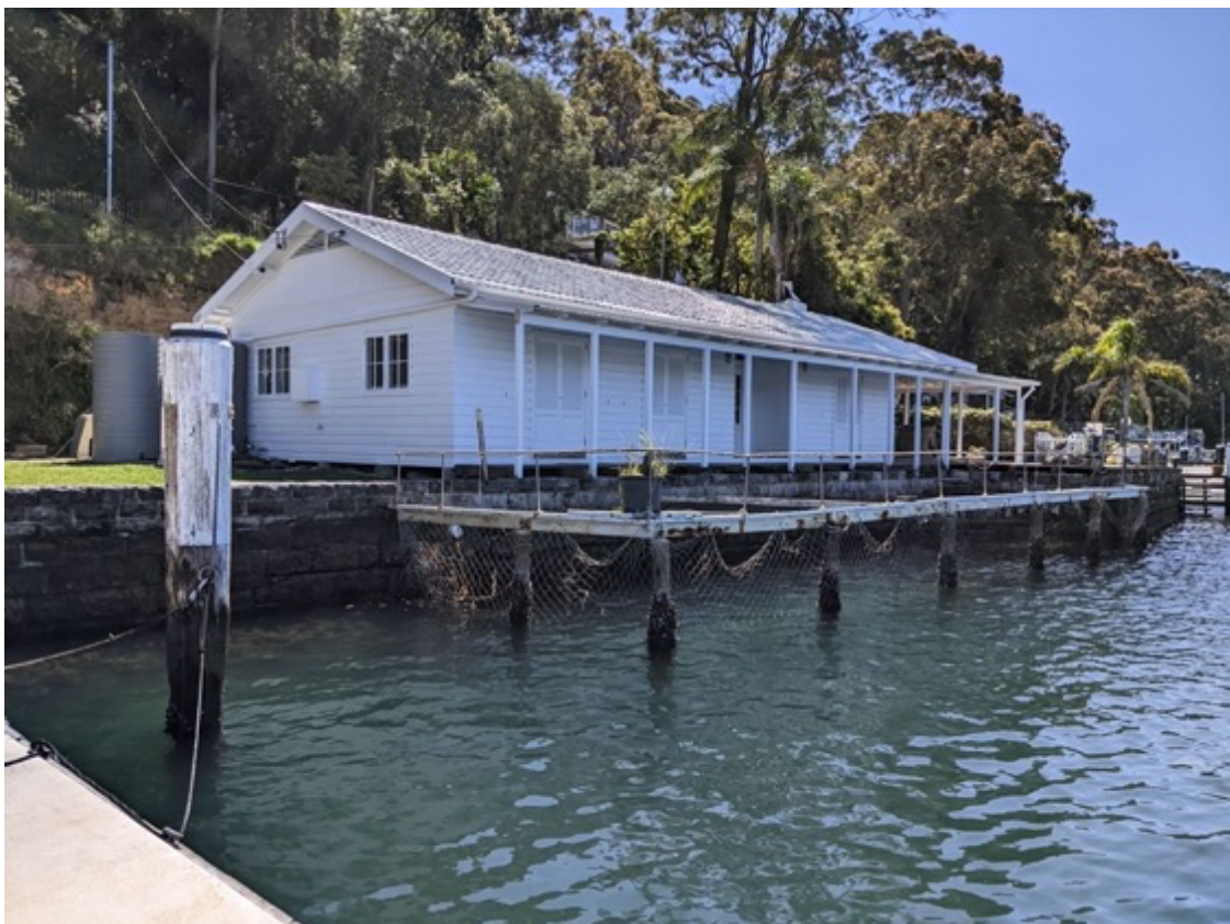
Figure 2 View of existing sea-pool facility, looking north-east. The riparian edge at this property comprises a block sandstone seawall with a paved reclamation behind.
