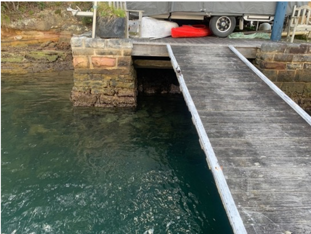
Figure 4 View of existing reclamation, seawall and ramp facility upstream of the sea pool facility, note intertidal oyster band on lower wall.
