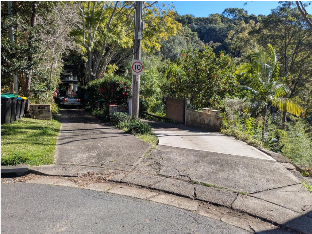
Fig 2: View of the existing driveway access to the subject site (RHS of view), No 4 Taminga Street and serving only one other property, No 4A Taminga Street (aka 55 Kananook Avenue), together with the independent driveway access to No 5 Taminga Street (LHS of view)
