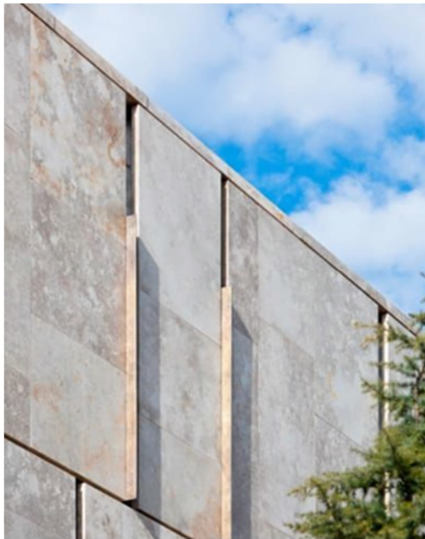
Figure 10- stone cladding
