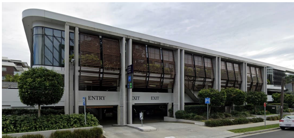
Figure 15-Existing Clarence Ave concrete blades with screen infills
