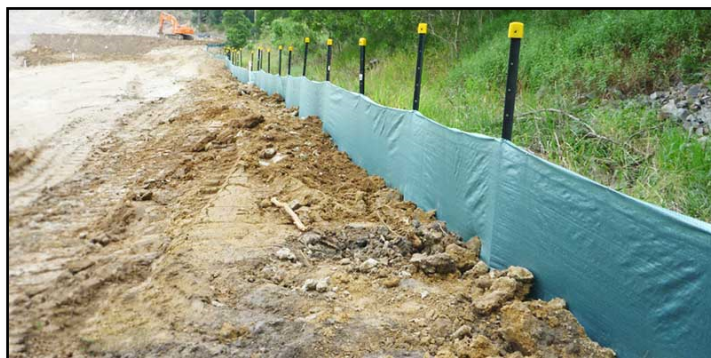
Figure 3: Sediment Fence
