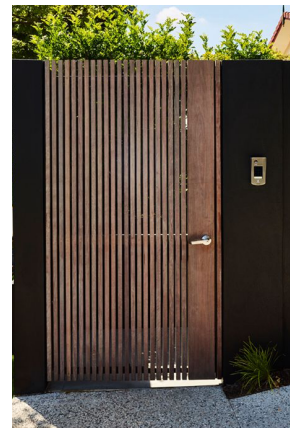
Vertical timber battens: front fence infill & gates
