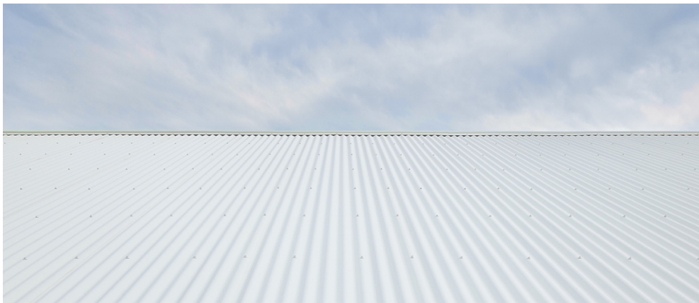
Roofing: custom orb profiled metal sheeting to match existing NCC classification 'light' to 'medium'
