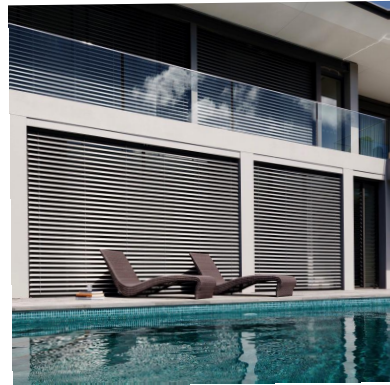
ANODISED ALUMINIUM WINDOWS AND EXTERNAL LOUVRES
