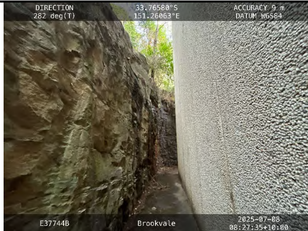
Photograph 1: Sandstone cut face observed along the eastern site boundary
