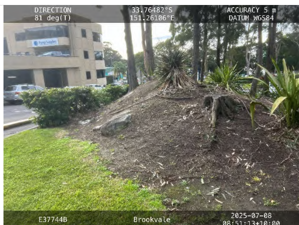
Photograph 3: Fill mound located along the northern site boundary
