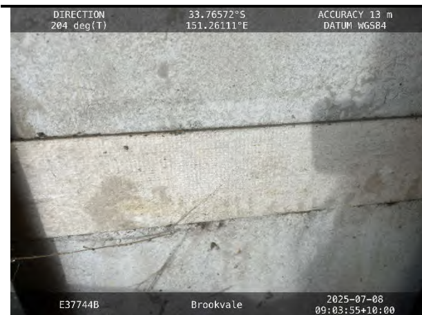
Photograph 4: Suspected asbestos containing internal cladding and joining panel
