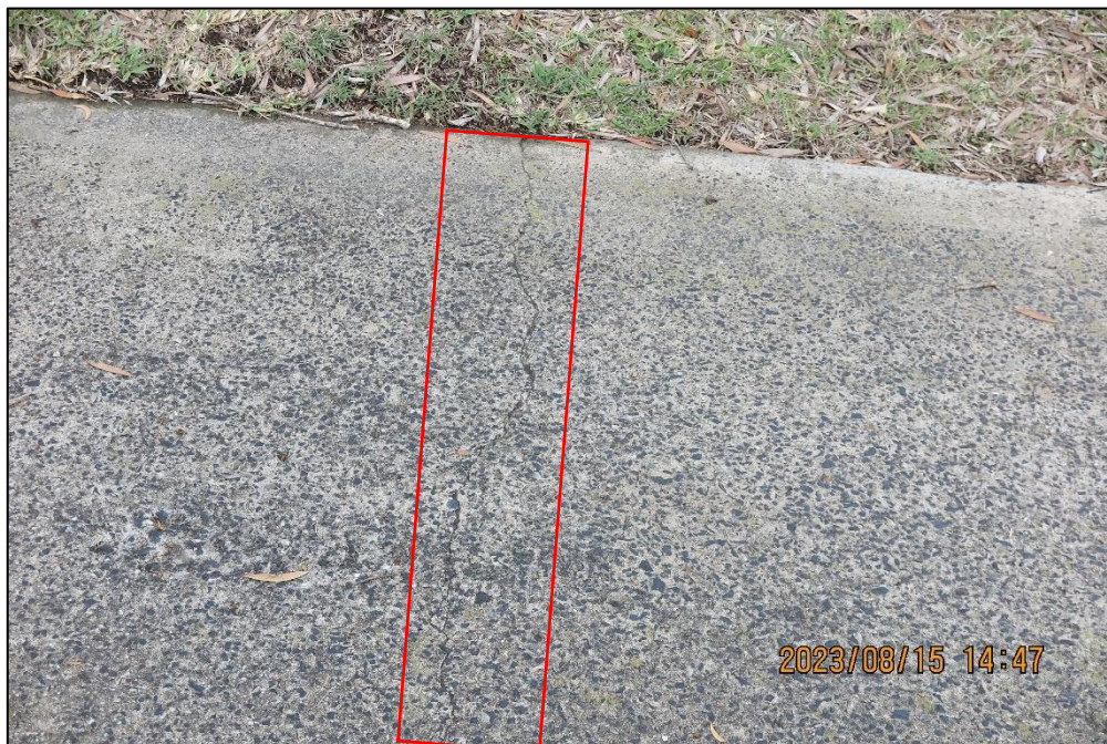
FIGURE 8: INSIDE THE RED RECTANGLE IS THE WITHIN TREE #6 SRZ RADIAL DISTANCE CRACK TO EXISITNG DRIVEWAY CONCRETE SLAB
