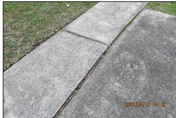
FIGURE 9: CONFIRMS DAMAGE AT THE TIME OF ASSESSEMENT TO BOTH THE CONCRETE DRIVEWAY SLAB AS WELL AS THE CONCRETE SIDE OF DRIVEWAY SLAB ADDED ON SECTION.
