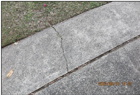
FIGURE 9: CONFIRMS DAMAGE AT THE TIME OF ASSESSEMENT TO BOTH THE CONCRETE DRIVEWAY SLAB AS WELL AS THE CONCRETE SIDE OF DRIVEWAY SLAB ADDED ON SECTION.
